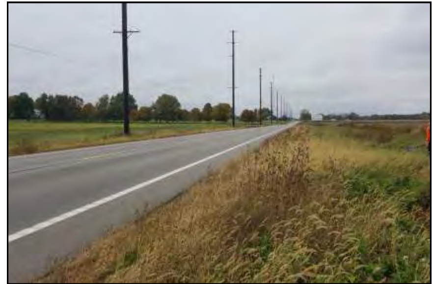
PS06, View Looking West
