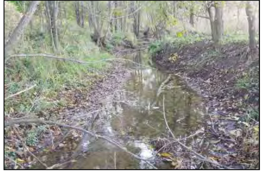
S03, View Looking Downstream
