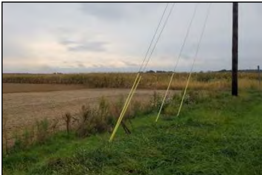
PS03, View Looking South
