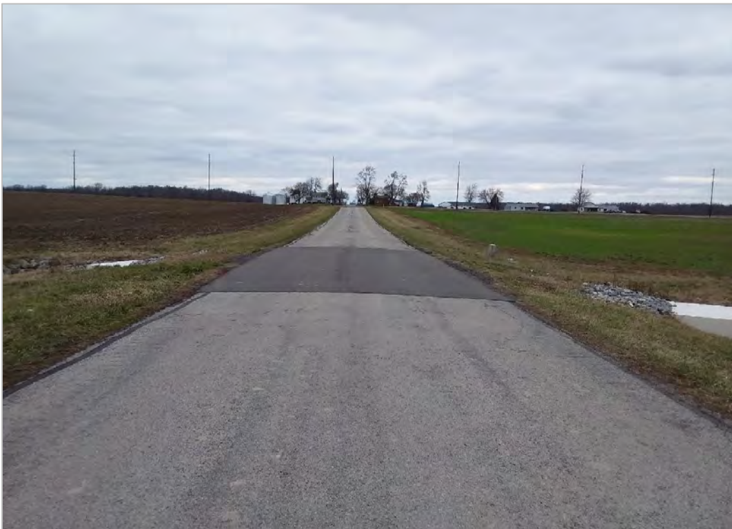
PHOTO 8: Pavement repair (patch) over concrete box culvert on CR22.
