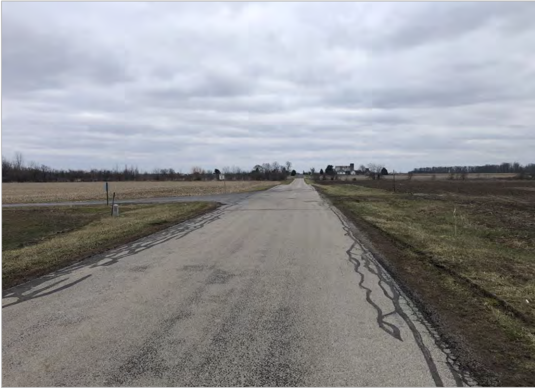
PHOTO 9: Intersection of CR22 and CR R, looking south.
