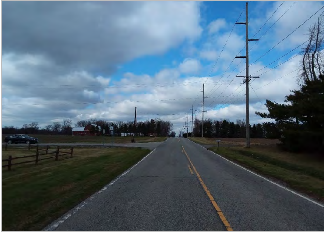
PHOTO 3: Intersection of CR23 and CR R, looking north.
