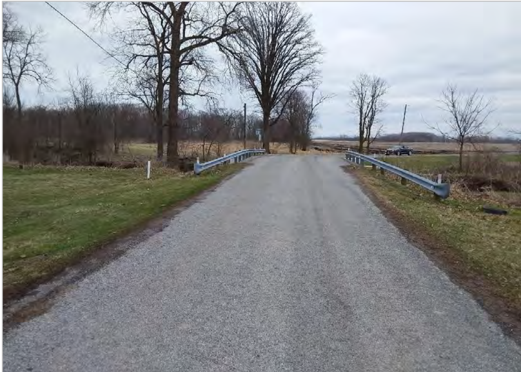
PHOTO 13: Bridge 2631717, looking east.
