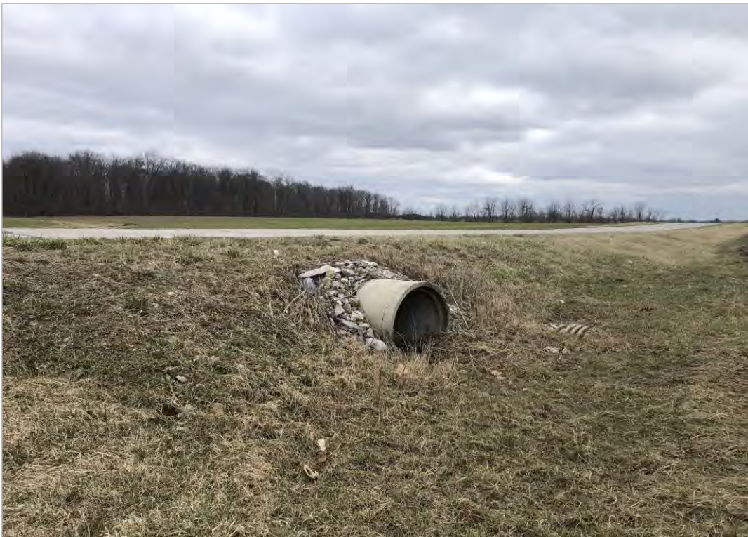
PHOTO 6: RCP culvert on CR22.
