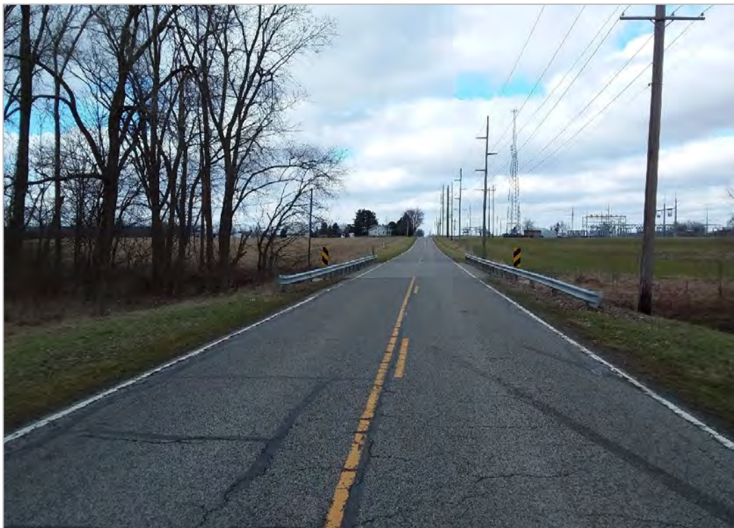
PHOTO 4: Bridge 2634821, looking north.
