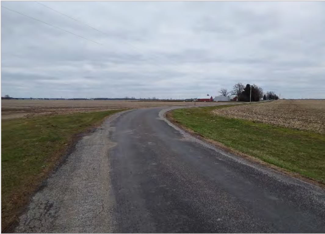
PHOTO 15: CR21-2 just east of Bridge 2631717, looking southeast.
