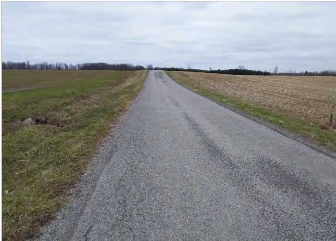
PHOTO 12: CMP culvert on CR R near CR 22.
