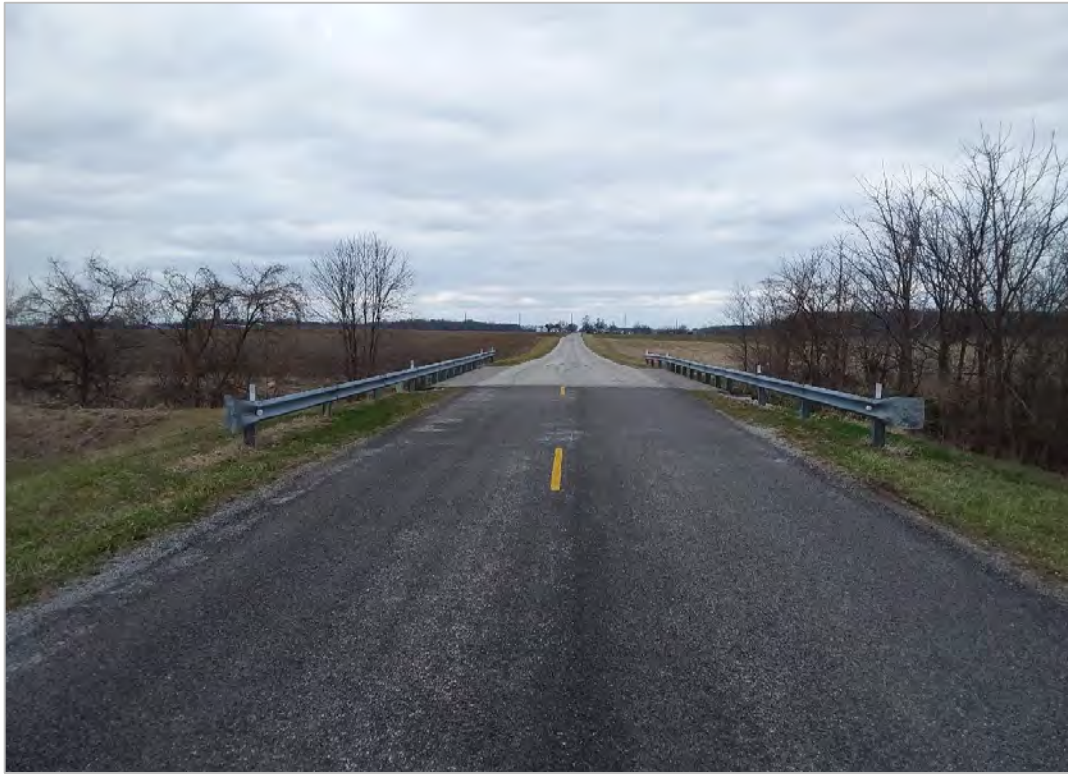
PHOTO 11: Bridge 2634732, looking north.
