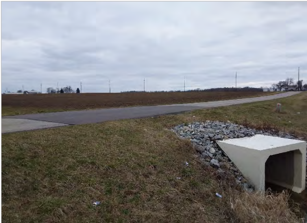
PHOTO 7: Concrete box culvert on CR22.
